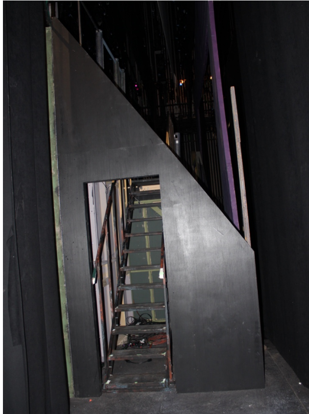
Figure 39: Backstage picture of the stud wall-jack-doorway supporting UGC platform
