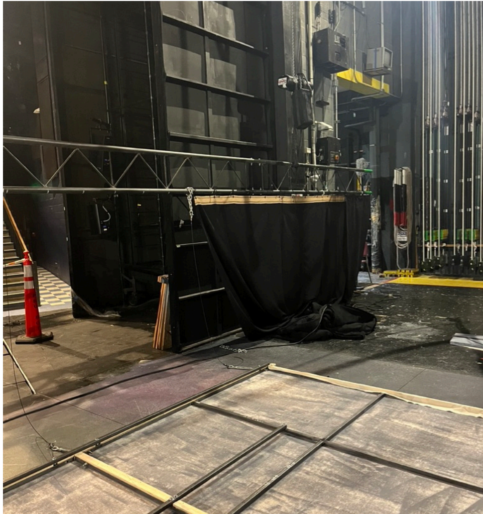
Figure 43: Proscenium Portal Load-in Process Photo – legs attached to truss batten
