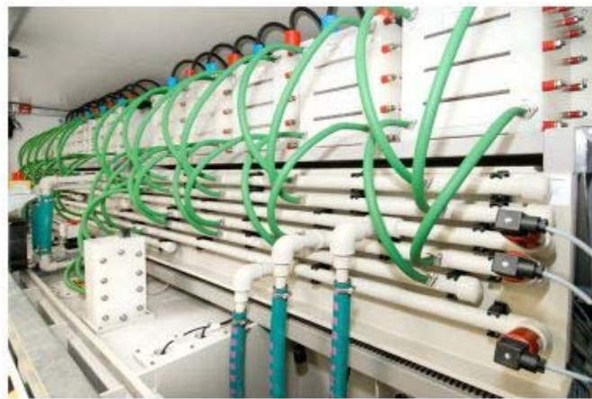
Figure 2-11: 100kWh Vanadium Battery System [37]
