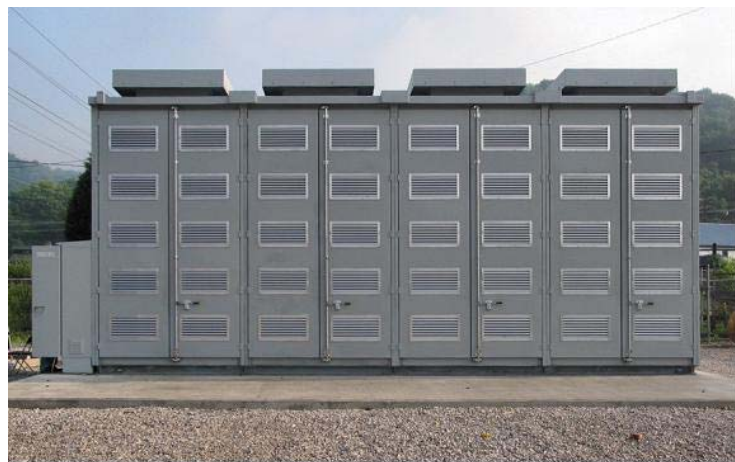
Figure 2-10: Safety Enclosure for NaS Battery [31]
