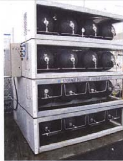
Figure 2-15: High Pressure Hydrogen Tanks [14]
