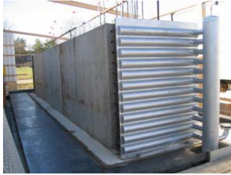
Figure 2-5: Concrete Thermal Storage [5]
