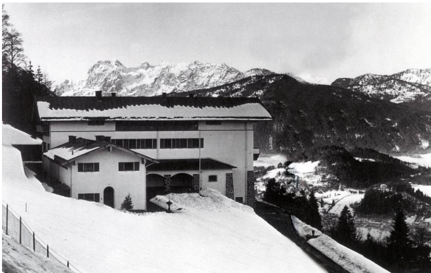
Figure 2-2. Berghof Exterior view.
