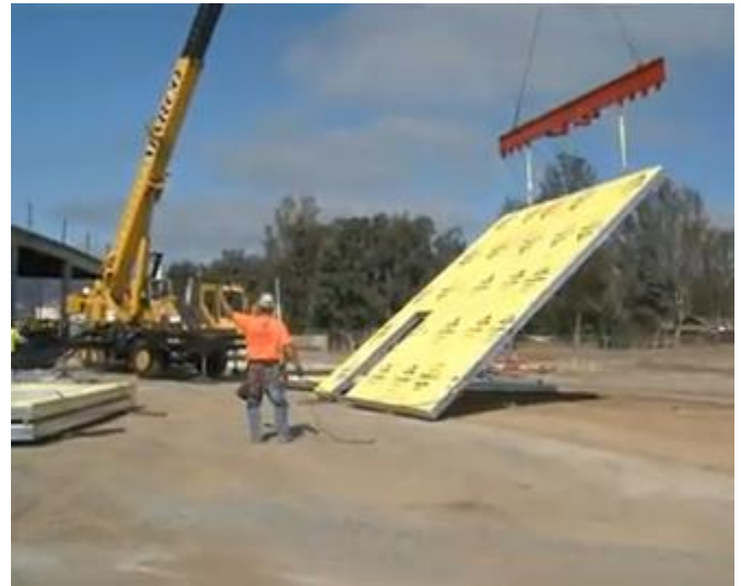
Figure 2.8: Partial Panel Prefabrication at Hospital in Temecula Valley, CA
