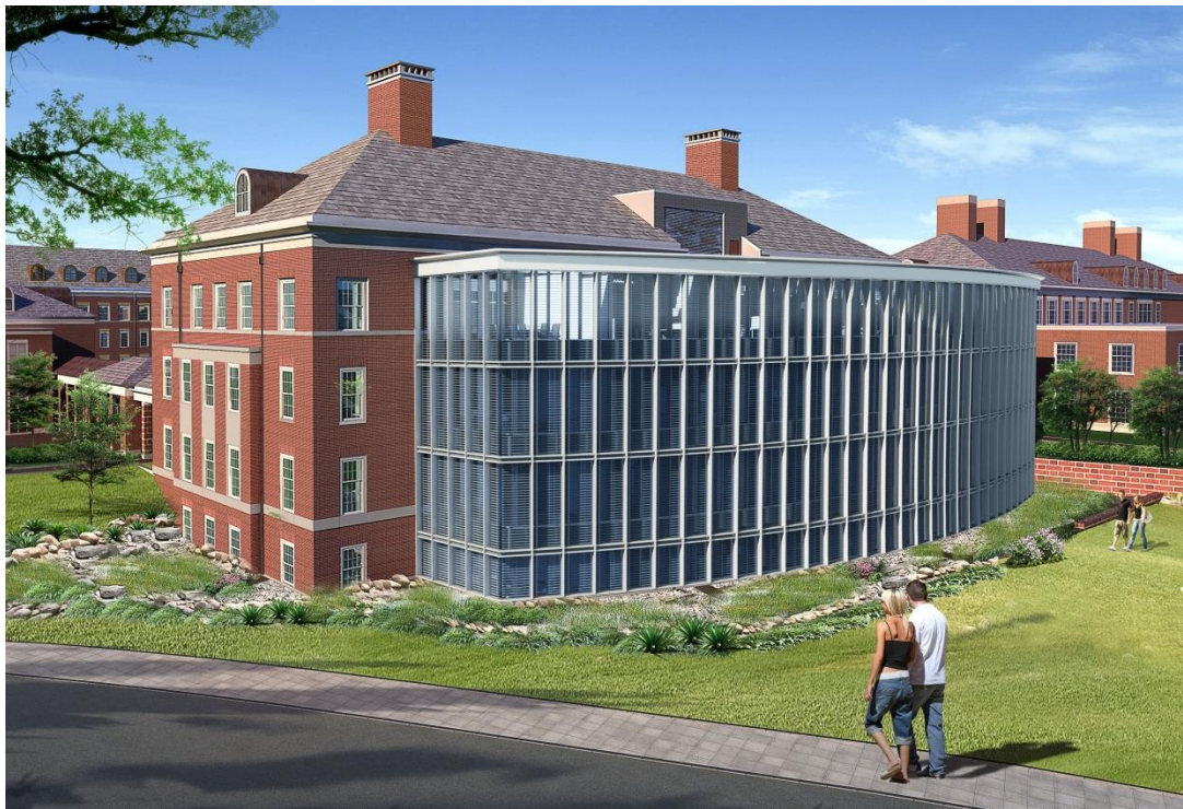
Figure 12 | URB East Facade with Double Skin Facade Redesign - Top image with operable louvers in raised position, bottom image with louvers lowered in horizontal orientation.
