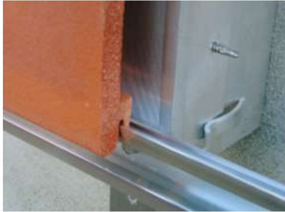
Figure 17: Panel Connection to Supports
