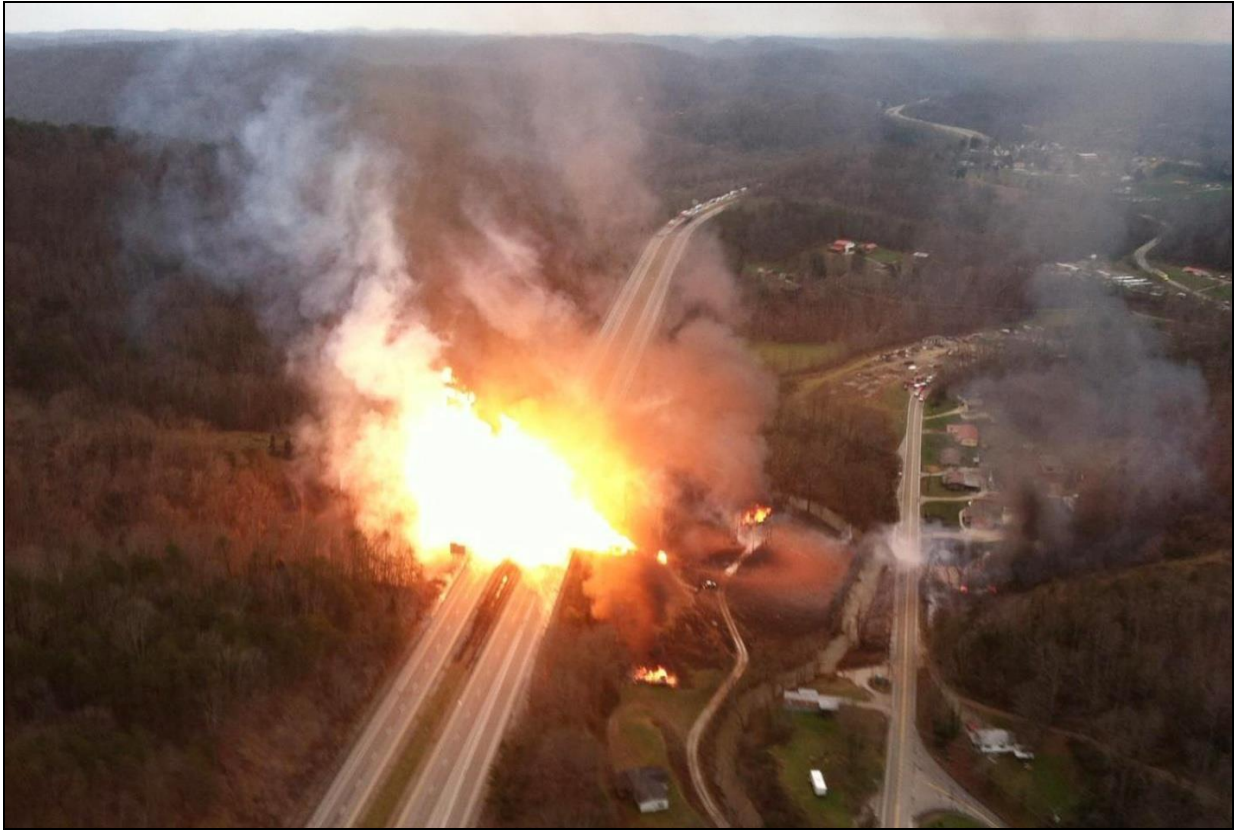
Figure 1: The explosion of a 30 inch natural gas pipeline in Sissonville, West Virginia on December 11, 2012 destroyed several homes and damaged Interstate 77. Amazingly, no one was killed. The National Transportation Safety Board (NTSB) determined that the pipe failure was due to external corrosion and lack of inspections [5].
