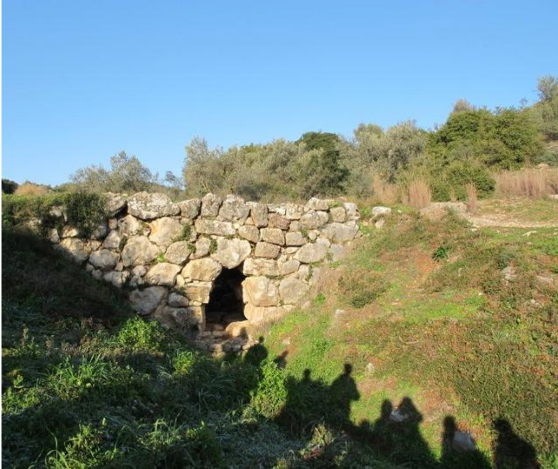
Figure 3. Example of Cyclopean masonry on a Mycenaean bridge. Photo by Katherine Burlingame
