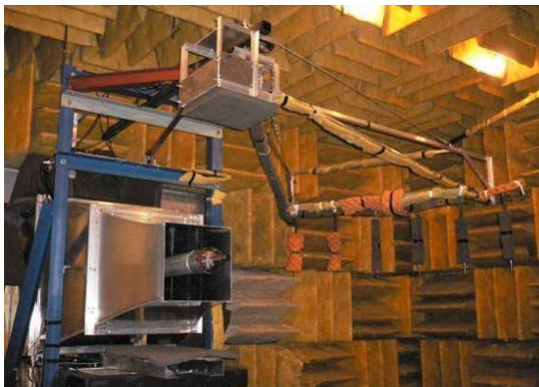
Figure 2-2. Photograph of the Plenum and Microphone Array
