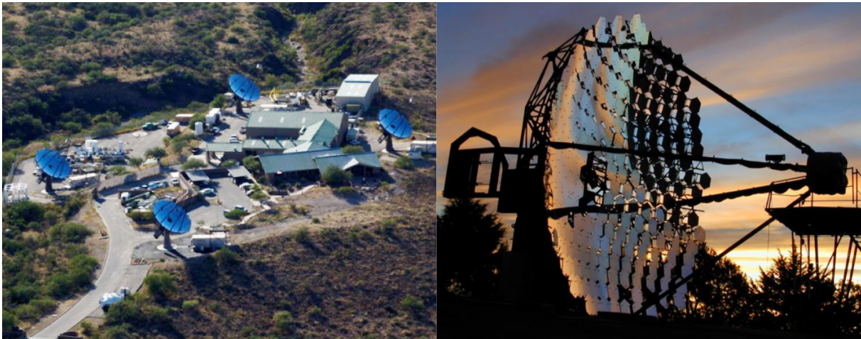
Figure 1.6: The four 12-meter Cherenkov telescopes that comprise VERITAS (left) [17]. Close-up of one of VERITAS's four Cherenkov telescopes with 350 hexagonal spherical mirrors (right) [18].
