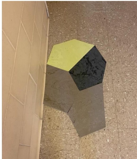
Figure 4: Verification of Repeating Pattern Alignment with Sample Tiles
