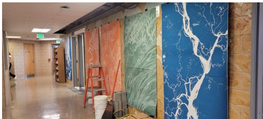
Figure 1: Printed Panel Designs during Hallway Renovation
